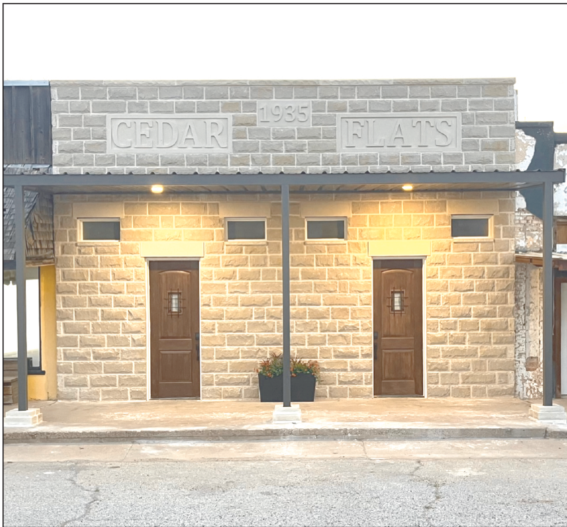
Downtown! Robert Lee is also seeing some changes being made to their downtown area. One of the historic buildings on Austin Street has been completely renovated into a beautiful new lodging establishment. The building, named Cedar Flats, has been converted into two suites and is available now for anyone needing a cozy place to stay in Robert Lee. For more information or to make a reservation, visit www.cedarflatstx.com .
