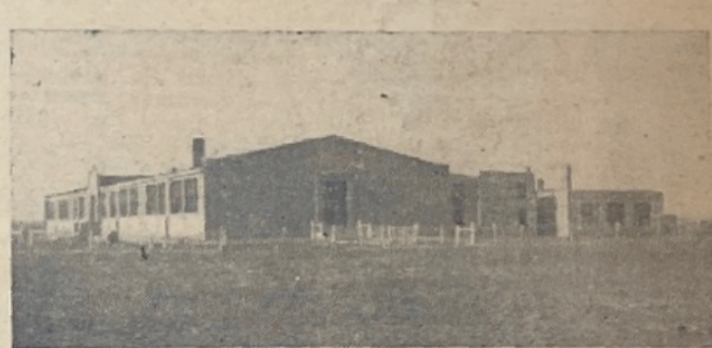
BLACKWELL SCHOOL BUILDING
